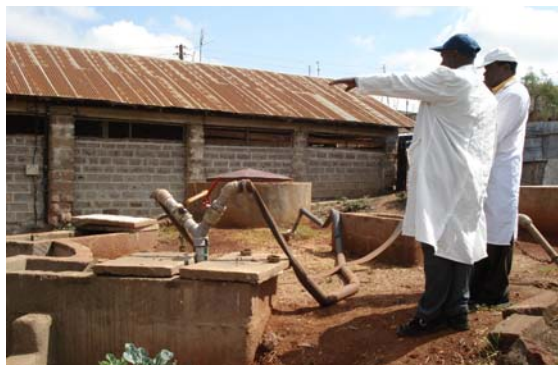
The contractor Paul Kariuki shows the biogas plant to Churchill Amatha
