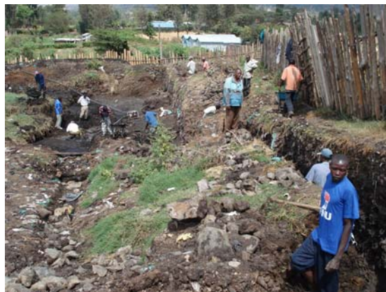
Work on the filtration ponds which must be finished by 20 th September 2008.
