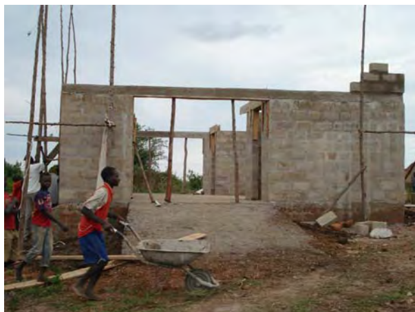
The new Gweri marketing collection centre which will house the cooler
