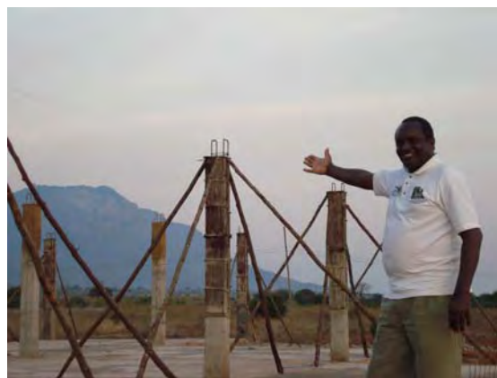
The market centre being constructed in Mwangaza
