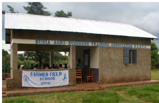
One of our multi purpose buildings
